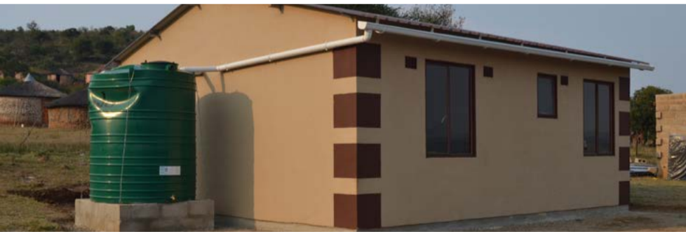
Enye yezindlu emsebenzini wokwakha iMsinga Top Rural Housing kaR44 million, enezindlu ezingu-300 eSigabeni sokuqala. Lo msebenzi ukuMasipala Wendawo uMsinga kanti uyingxenyi yohlelo lukahulumeni wesifundazwe ekuthuthukiseni ingqalasizinda yezindlu nezindawo zokuhlala eSifundeni uMzinyathi.
